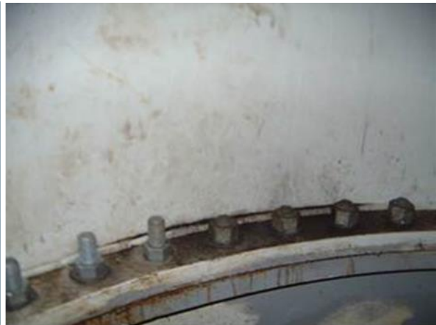
Crack in the weld of the flange to the tower
